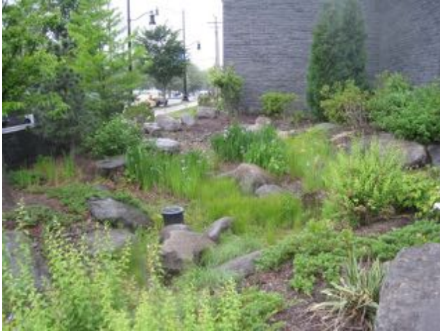
An exemplary display of green infrastructure at The Commonwealth Medical College in the City of Scranton.
