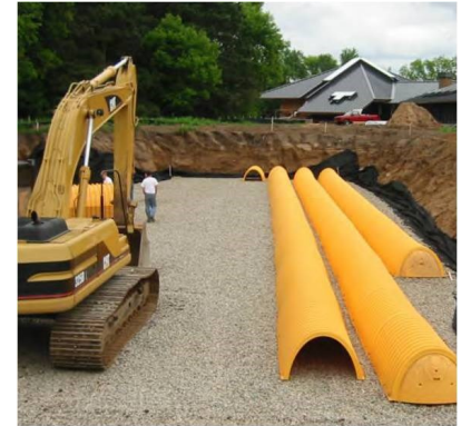
Volume control BMPs modeled for the high-density TOD stormwater management plan included rainwater harvesting (above left), below-ground recharge systems (above), and green roofs (left).
