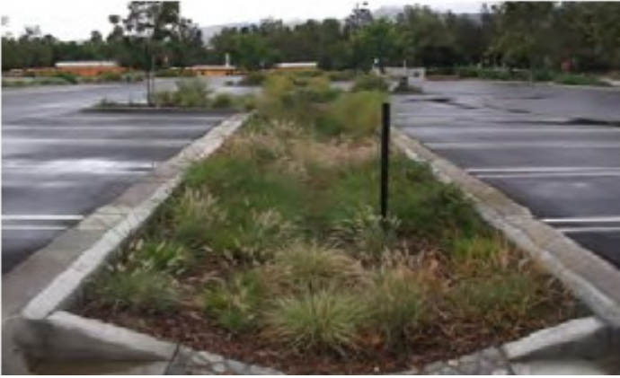
Bio-retention (rain garden) installation.
