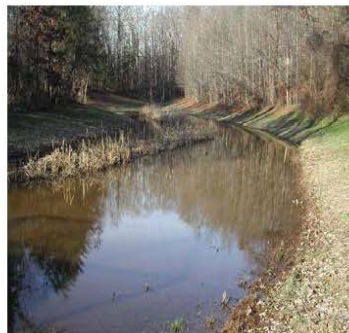
Stormwater pond at Northridge
