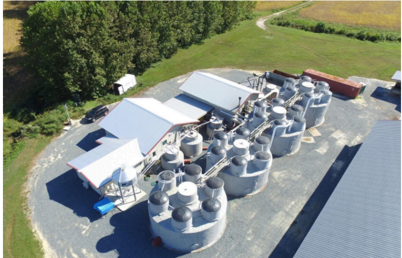
Figure 5. Planet Found Energy Development's anaerobic digestion and nutrient capture system at Millennium Farm. Credit: PFED.
