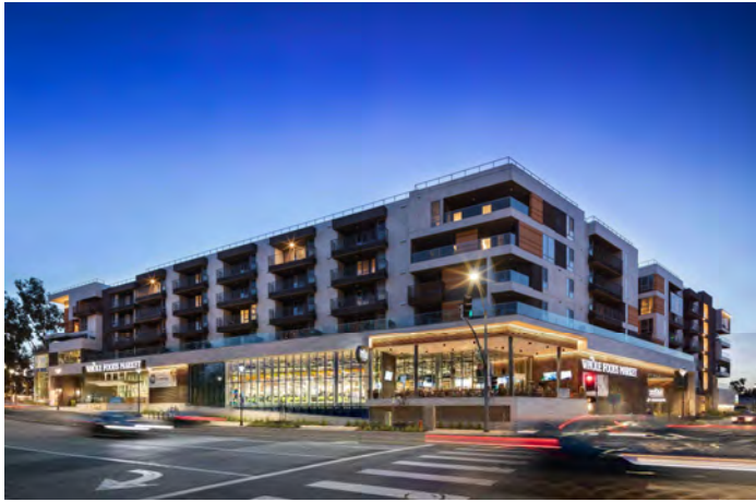
A view of Whole Foods Market on the lower section and Talaria residential above.
