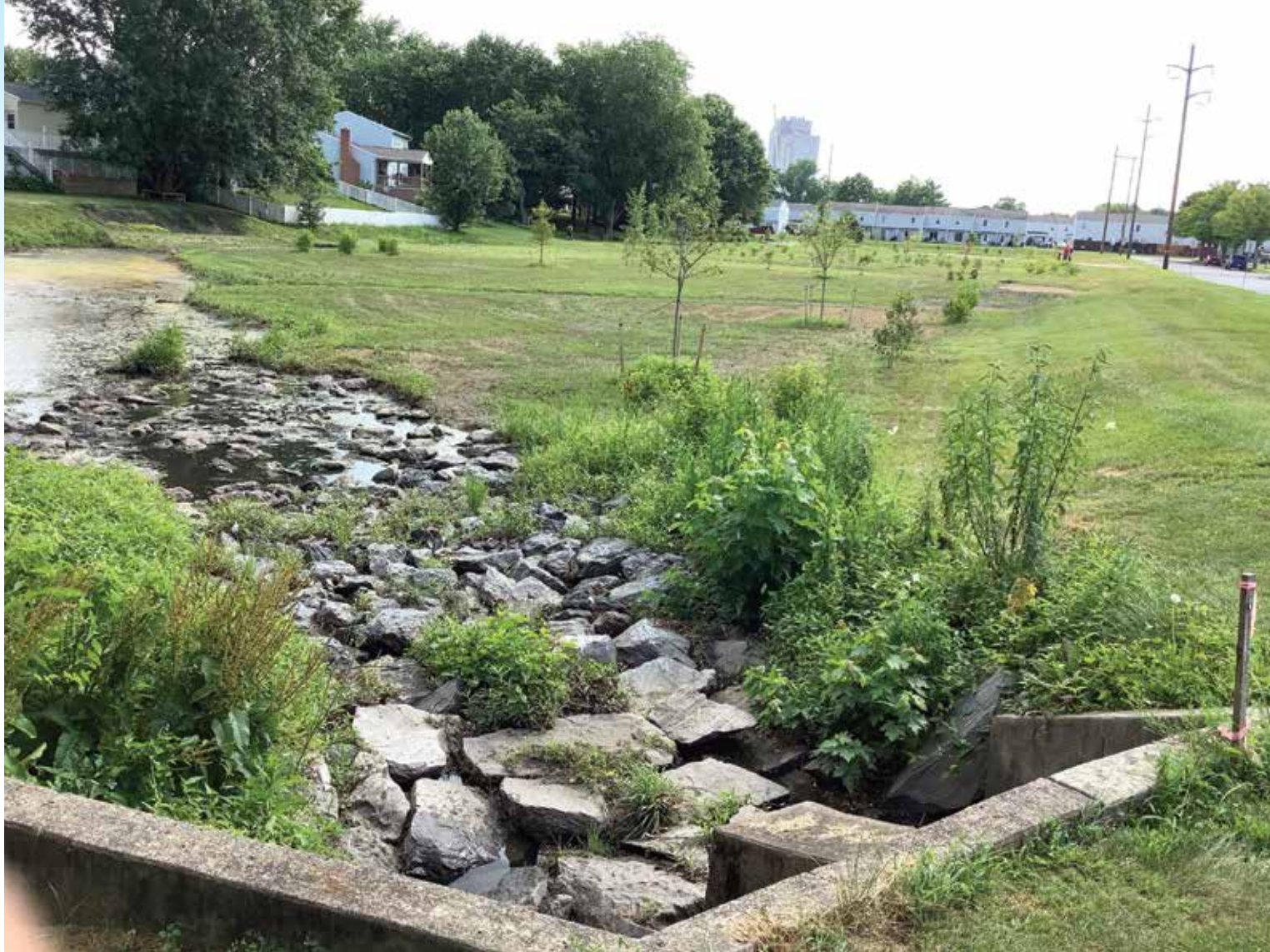
Retro-fitted basin constructed by the Mechanicsburg Borough captures drain from downtown and residential sectors.
