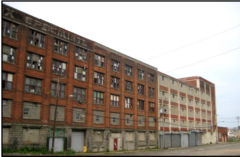
Figure 4: 500 Seneca St., before redevelopment. Source: CJS Architects LLP
