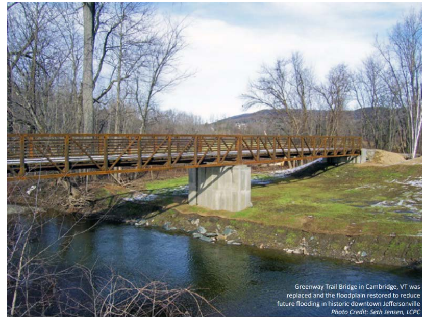
Greenway Trail Bridge in Cambridge, VT
