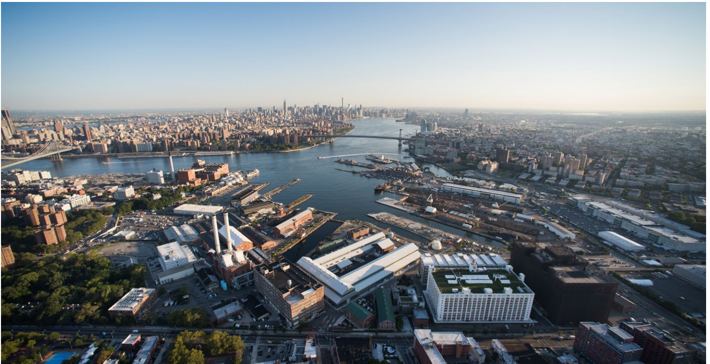
Brooklyn Navy Yard were decommissioned and changed to be a industrial site focusing on light manufacturing and technology.
