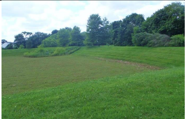
Looking south at outfall structure
