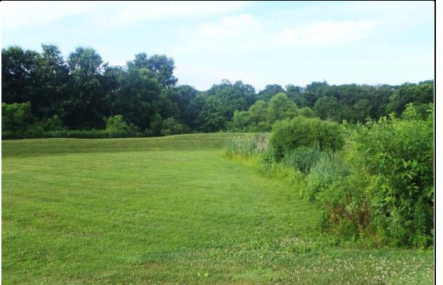
17E Dry detention looking south towards control structure
