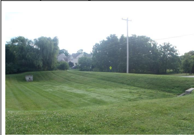
Typical Dry detention area
