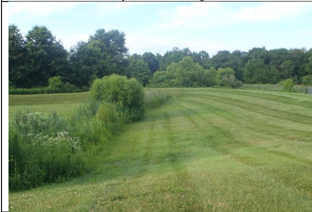
17E Dry detention looking south towards control structure
