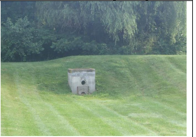
Typical Control Structure
