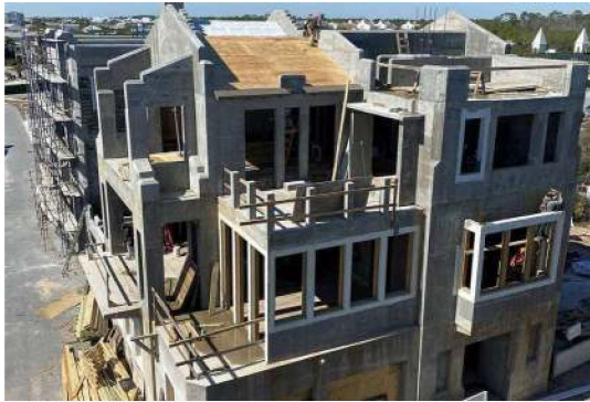
Figure 22: Masonry block construction, one component of the FORTIFIED system..
