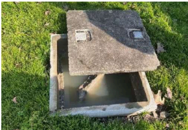
SEPTIC TANK ACCESS HATCH SHOWING HIGH LIQUID LEVEL
