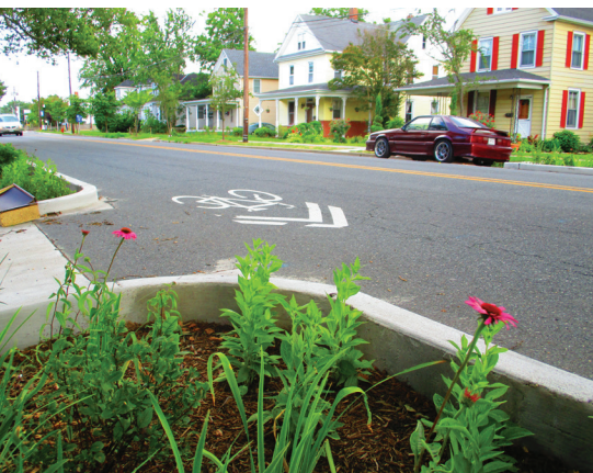
A rain garden in a sharrow in Cambridge Md. Photo: Mike Hunninghake.
