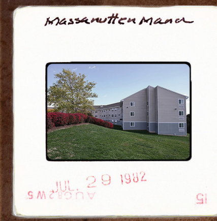
(L to R): St. Bartholomew’s House, Bethesda, Md.; Kirkwood House Senior Apartments, Baltimore, Md.; Massanutten Manor, Strasburg, Va. Architect: Bennett Frank McCarthy Architects. Slide photos: Ralph Bennett. Background: Alexander Dzurec, Autotroph.
