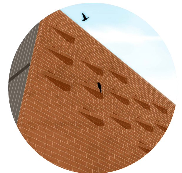
Two views of a high, horizontal band of bird boxes for nesting birds: the boxes are distributed in a running bond pattern that echoes the existing brick bond of the facade. Renderings: Emily Kelly.
