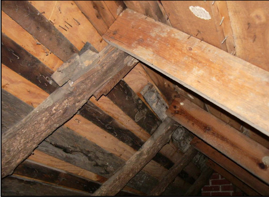
Figure 5. Original pole rafters butted and fastened to west side replacement rafters (2015).
