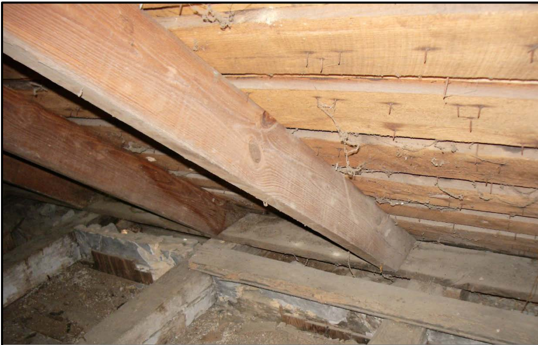
Figure 6. Replacement rafters, shingle lathe, and false plate on west side (2015).
