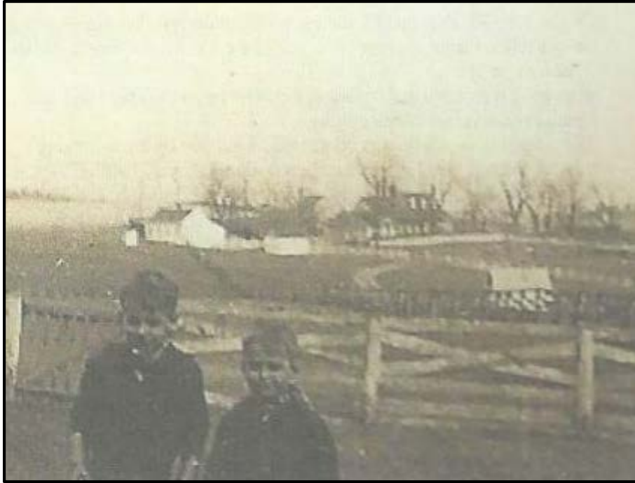
Figure 23. Royston family photograph (1941); former slave quarter viewed from the south, with full-length east porch, painted white, and surviving privy.
