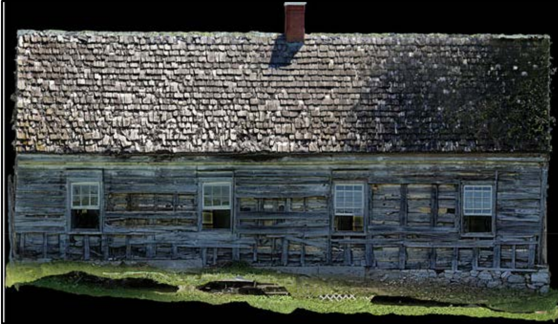
Figure 12. Slave quarter west wall (2015); all window openings have been widened 4”.
