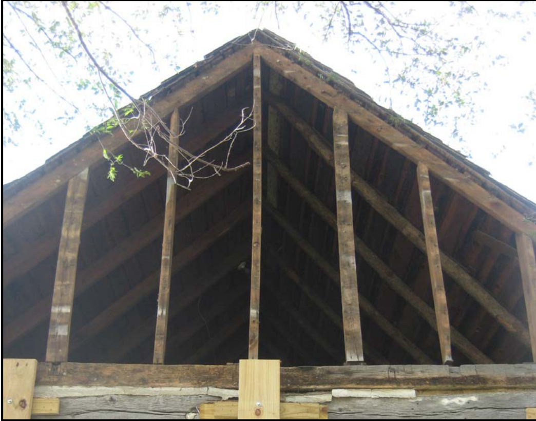
Figure 8. Slave quarter south gable with replacement end rafters and studs (2015).
