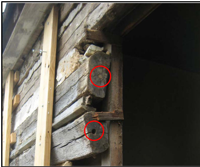
Figure 15. Slave quarter SW window opening (2015); holes for pegs in three side logs, one with sawed off remnant of peg.
