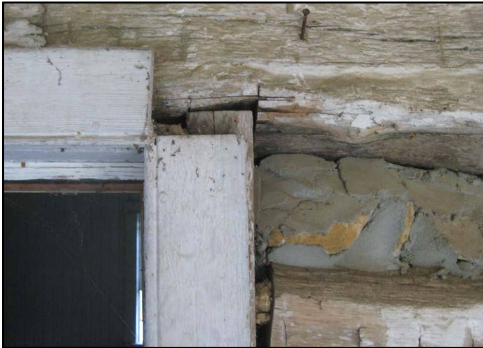
Figure 17. East façade detail (2015), notched jamb for original doorway.
