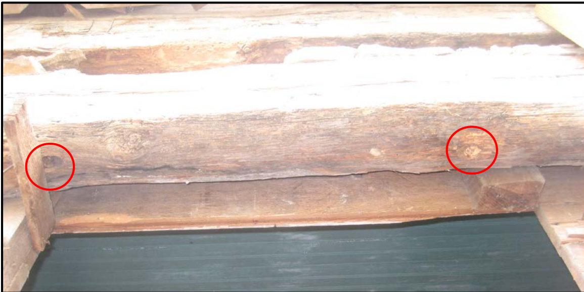
Figure 13. Slave quarter west wall, SW window (2015), cut-off pegs in top log of opening, cut stud and siding in room 504.
