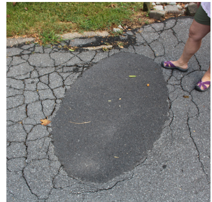
Figure 6 Repaired sinkhole at Glenwood Pool
