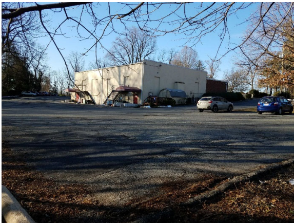
Figure 1: Bioretention opportunity downslope of a large parking lot
