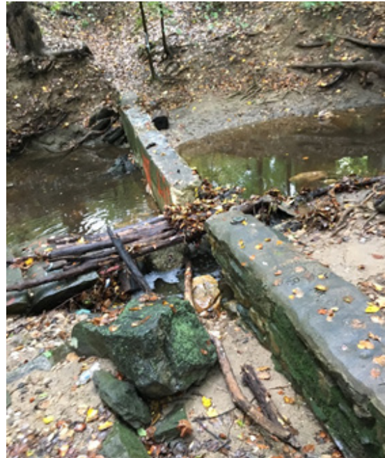
Exposed pipe in stream
