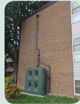
Cistern, Glenway Gardens
