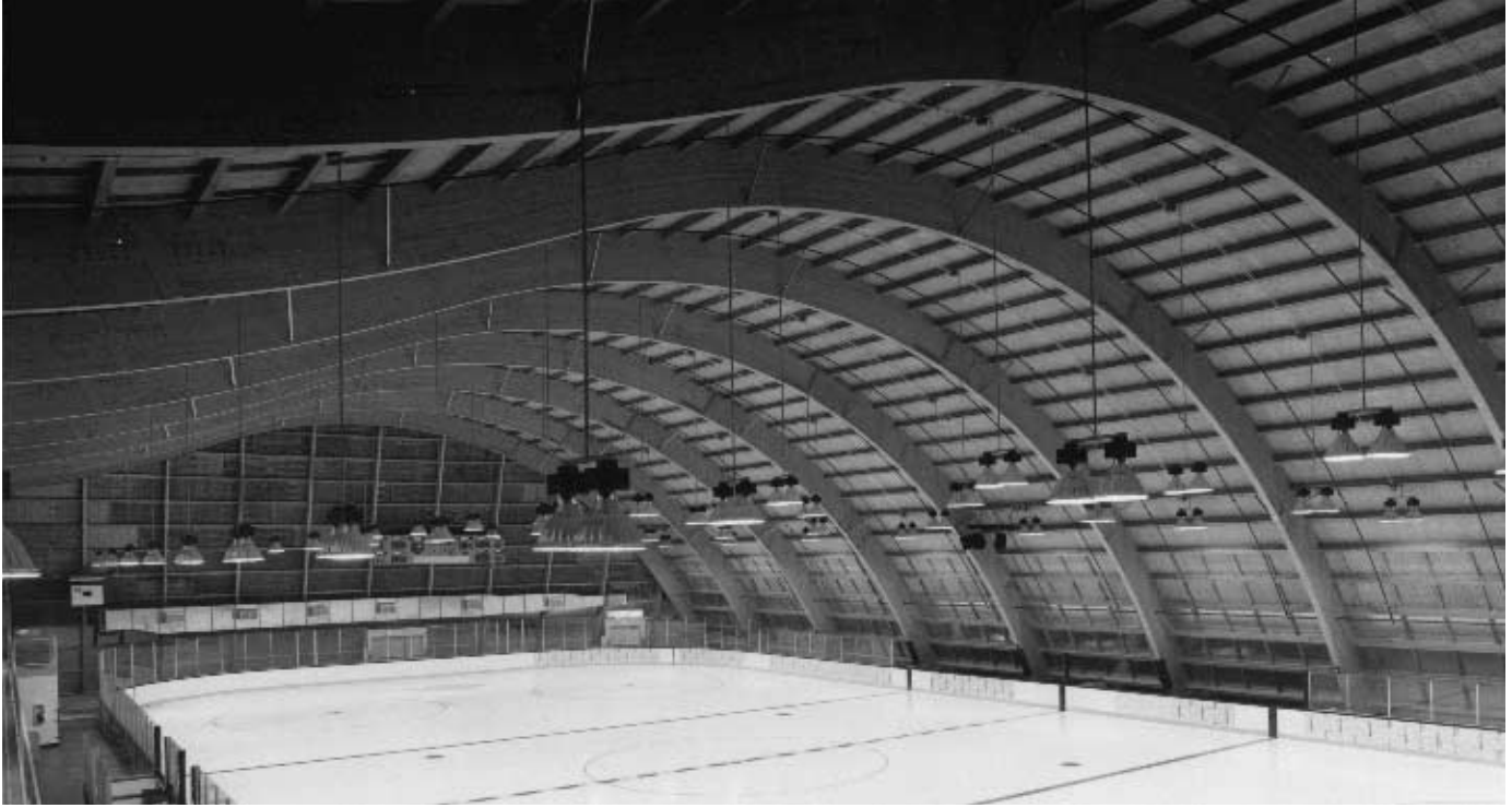
The Disney ICE rink in Anaheim, California features glulam arches curved to a 75-foot radius to form the ice center's roof system.
