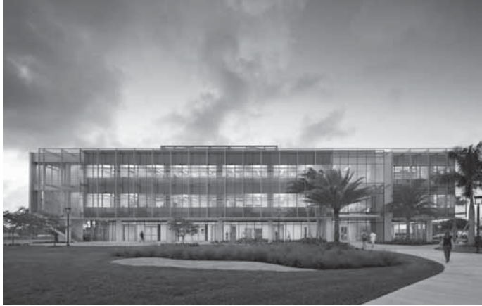
Ed LeBard (M.ARCH '02, B.S. Architecture '00) worked as a project architect on Lynn University International Center. The project collected a National AIA Institute Honor Award in 2015 and recently received the Gensler Design Excellence Award from Firmwide. (Photo Credit: ©Michael Moran/OTTO)
